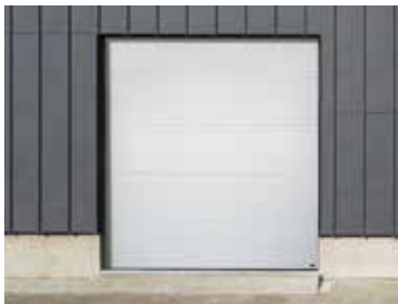
REPAIRED DOOR WITH AMARR 2747 REPLACEMENT SECTION
